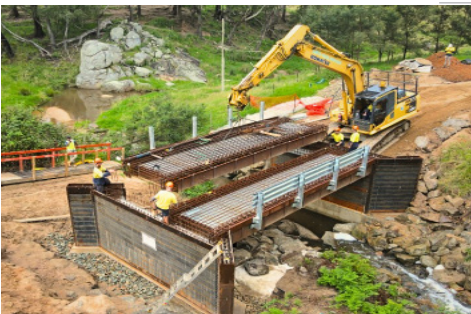
Single Span Bridge
