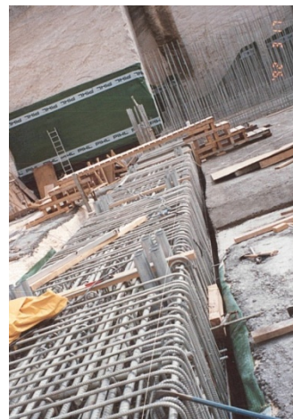
Figure 6. Heavily galvanized reinforced insitu beams for Tynes Bay.
