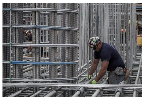
Figure 14. Installing galvanized reinforcement in the main span towers.
