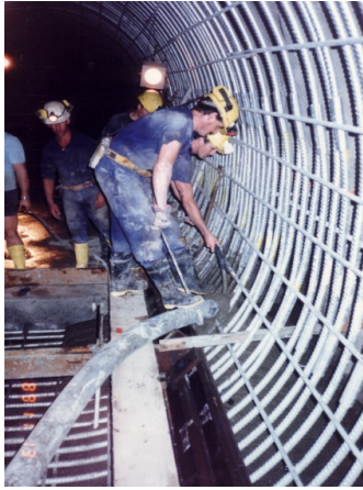
Figure 9. Sydney ocean outfall tunnels for treated effluent.
