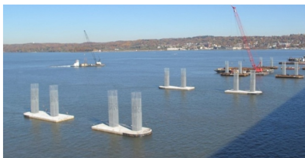
Figure 13. Galvanized reinforcement in approach spans of the new New York Bridge
