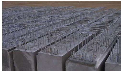
Figure 12. Precast galvanized reinforced sections for Denia Port.
