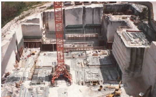
Figure 5. Foundations for the Tynes Bay Waste-to Energy Facility, Bermuda.
