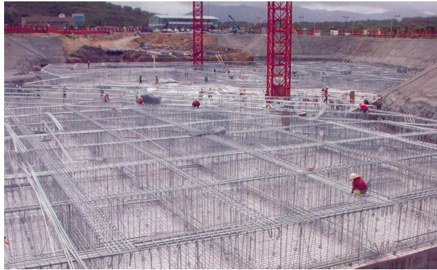
Figure 10. Foundations for National Museum of Marine Biology and Aquarium, Taiwan.
