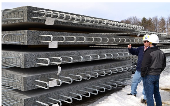
Figure 15. Galvanized reinforced precast bridge deck panels - New York Bridge
