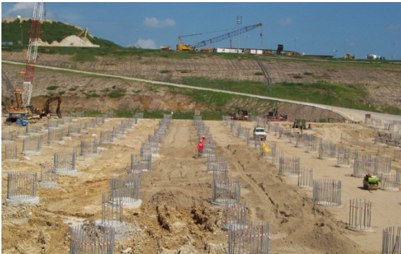
Figure 7. Galvanized reinforced foundation piles - Changi Water Treatment facility.
