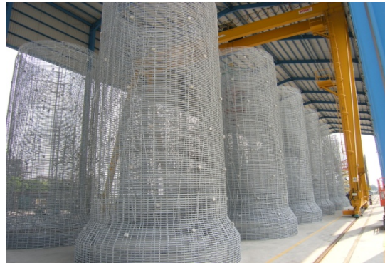
Figure 8. Prefabricated galvanized reinforced pipe cages for slip forming.
