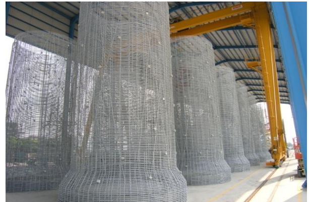
Figure 7. Prefabricated galvanized reinforced pipe cages ready for slip forming.
