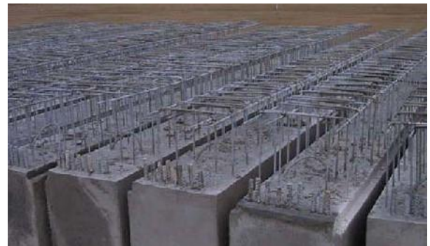
Figure 8. Precast galvanized reinforced seawall sections for Denia Port, Spain.
