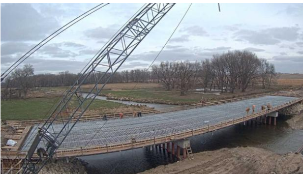
Figure 6. Continuously galvanized reinforcement in the Buffalo Creek Bridge, Independence, Iowa.
